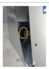
• Push the plastic tube through the hole in the baseplate, and the hose clamp. Then push the tube over the nipple on the condensate tray.
